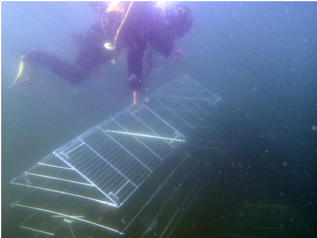
Fig. 5: Installation of enclosure.
